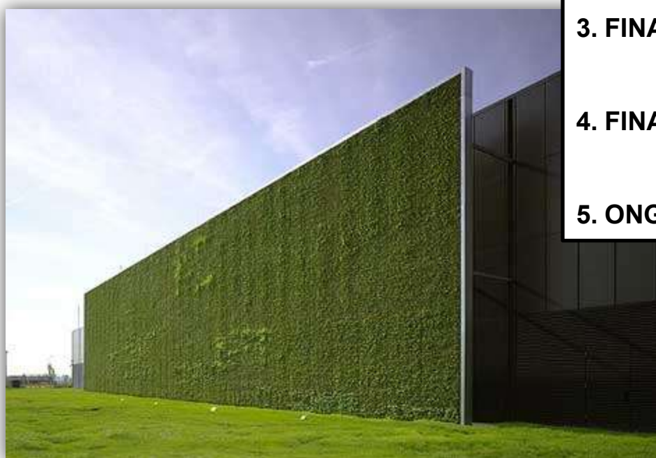
Fig 24.1. – Green wall at Citi Data Center in Frankfurt German Data Center
